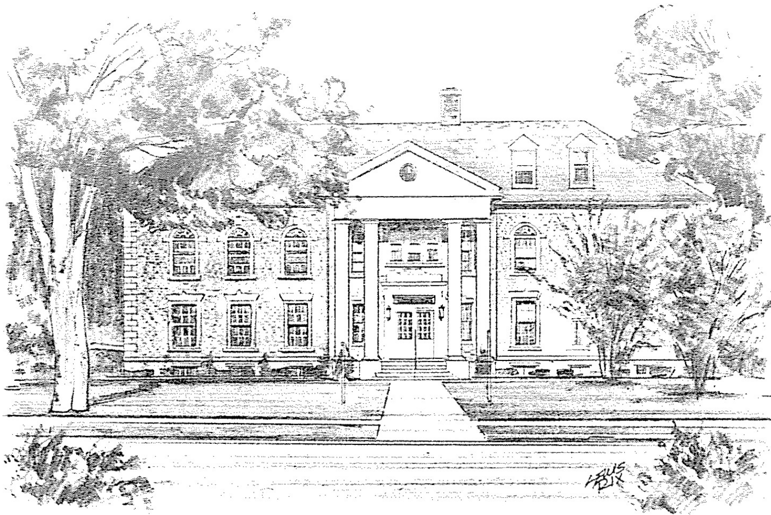
Wyoming County Court House Warsaw, New York
